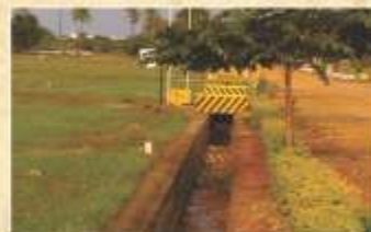
Storm Water Drain
